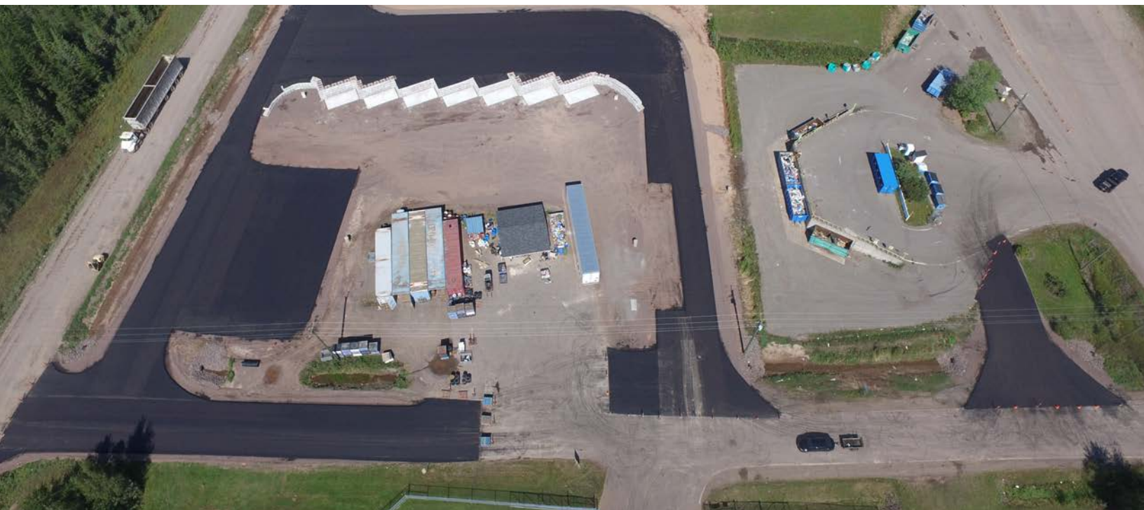
Figure 1: New Public Drop-off Construction
