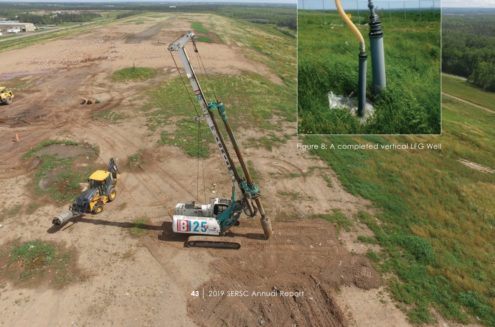
Figure 7: Drilling of a Vertical LFG Well
