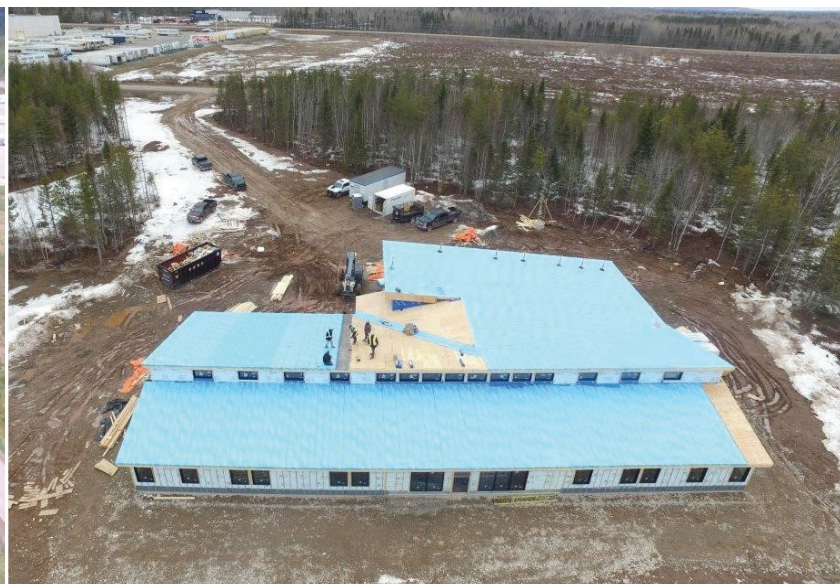
Figure 3: New Administration Building Under Construction
