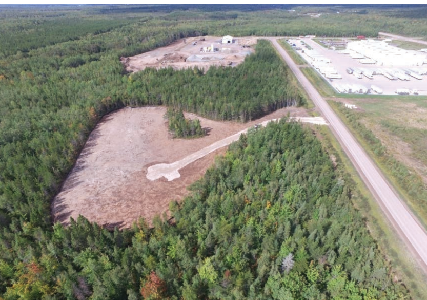
Figure 2: Site Clearing for New Administration Building
