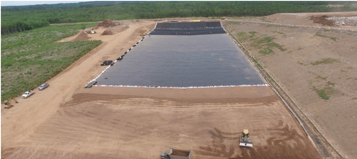
Figure 9: Liner Placement during Cell #16 Construction
