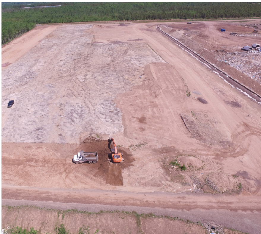
Figure 3: Pre-excavation of Cell 17
