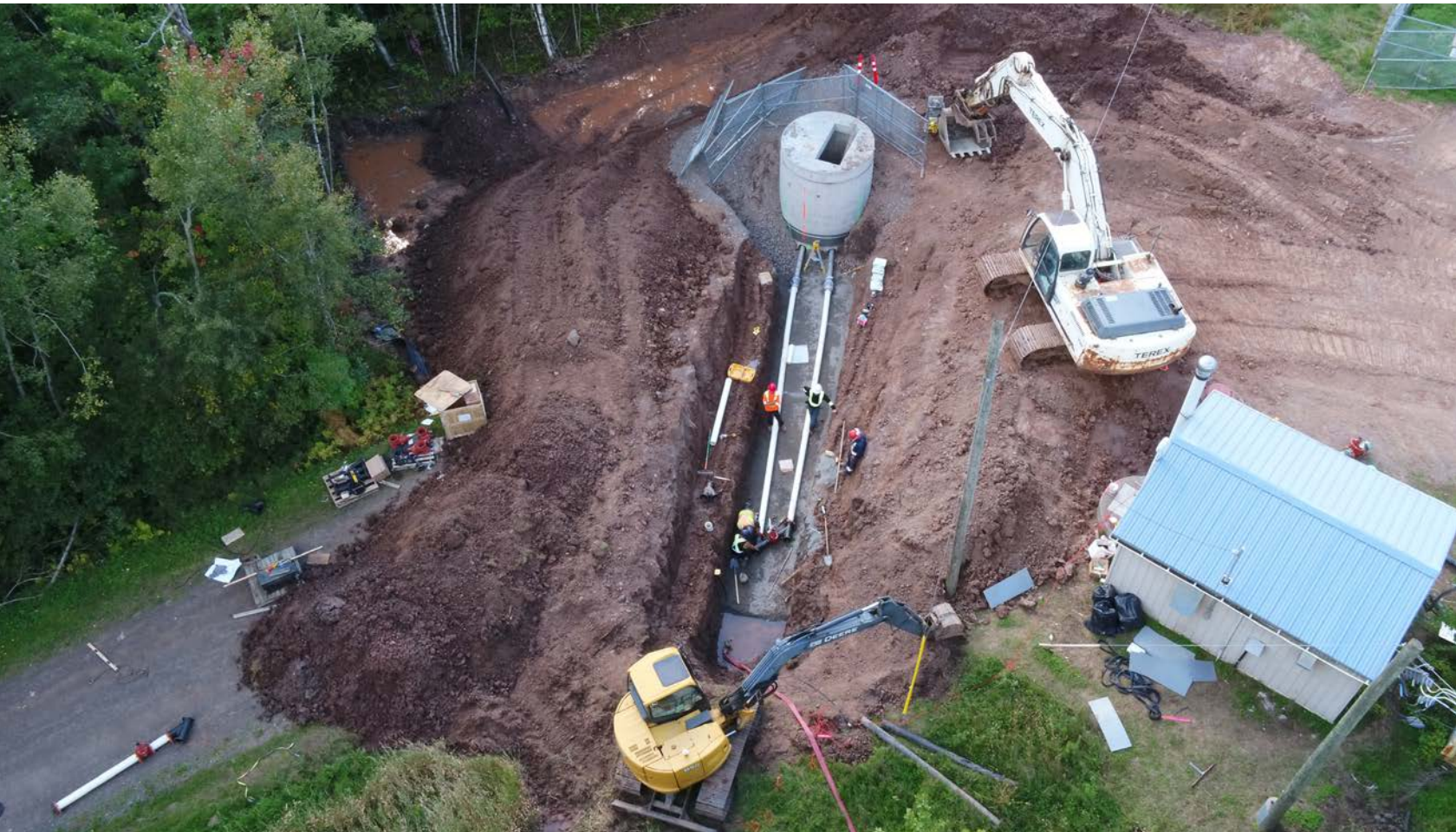
Figure 1: Construction of the leachate effluent pump station
