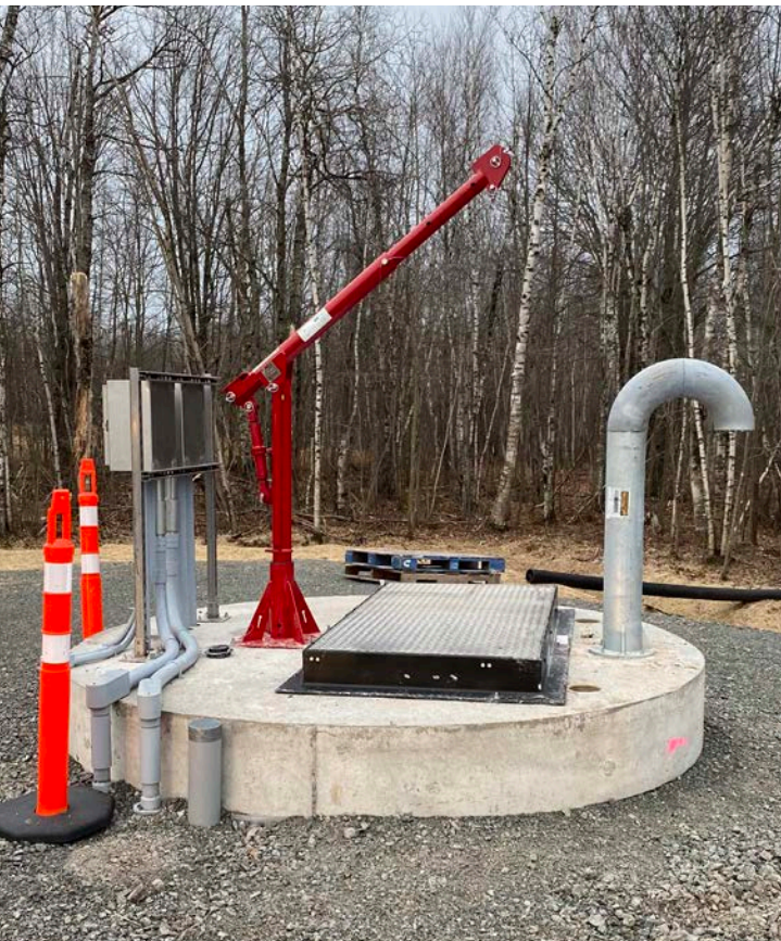
Figure 2: Completed leachate effluent pump station
